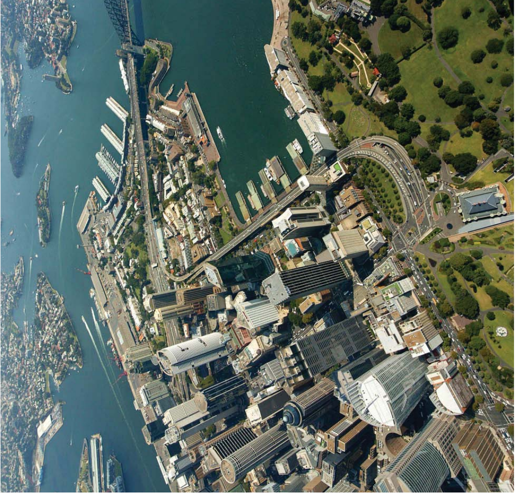
Aerial view of the precinct in the context of the Sydney CBD
